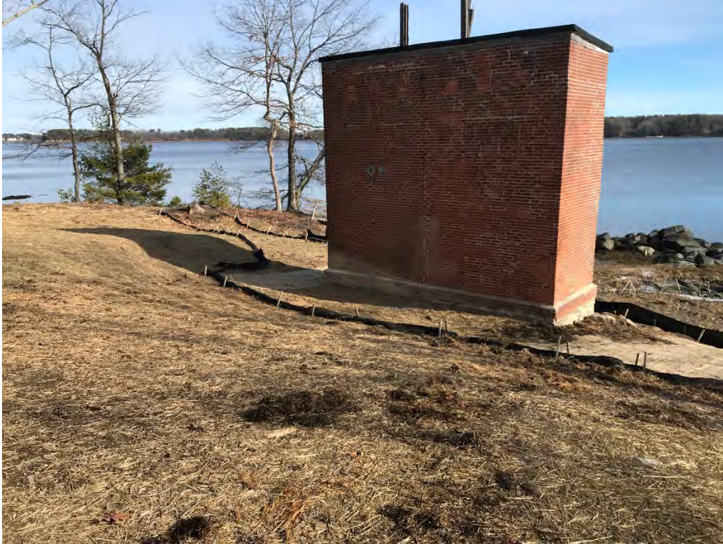
Fig 1: Slope leading down to cable house and salt marsh restoration at the Eversource property/west side of the bay. Viewing northeast. (01-19-21)
