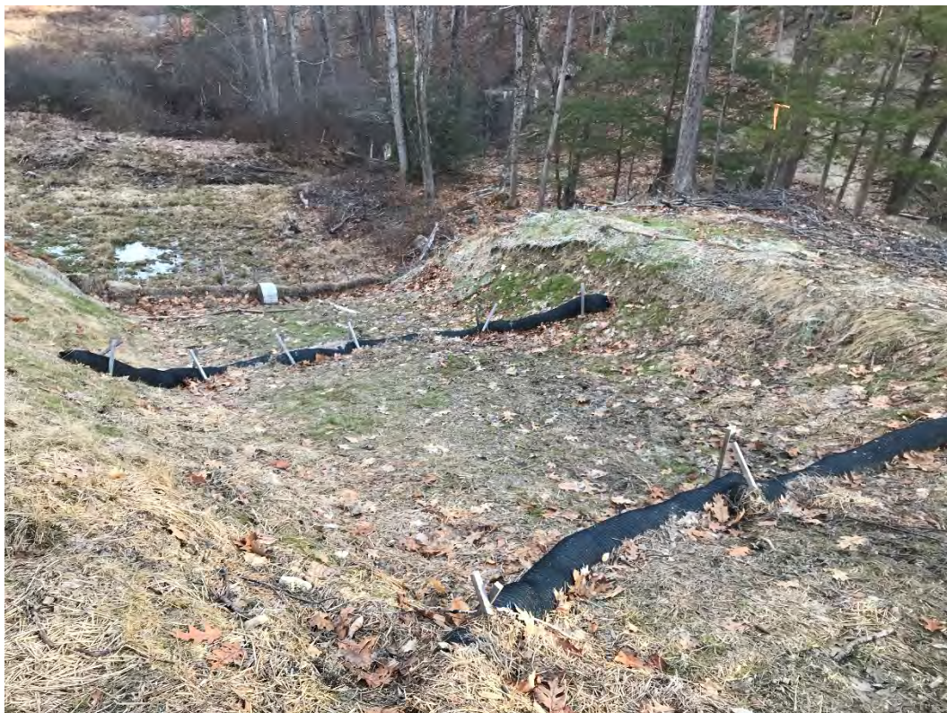
Fig 7: Lower portion of slope between Strs. 28 and 29. Viewing northeast. (01-19-21)
