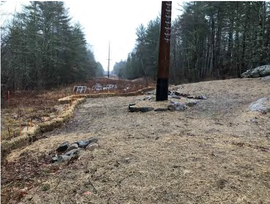
Fig 3: Str. 89 work area. Viewing southeast. (01-16-21)
