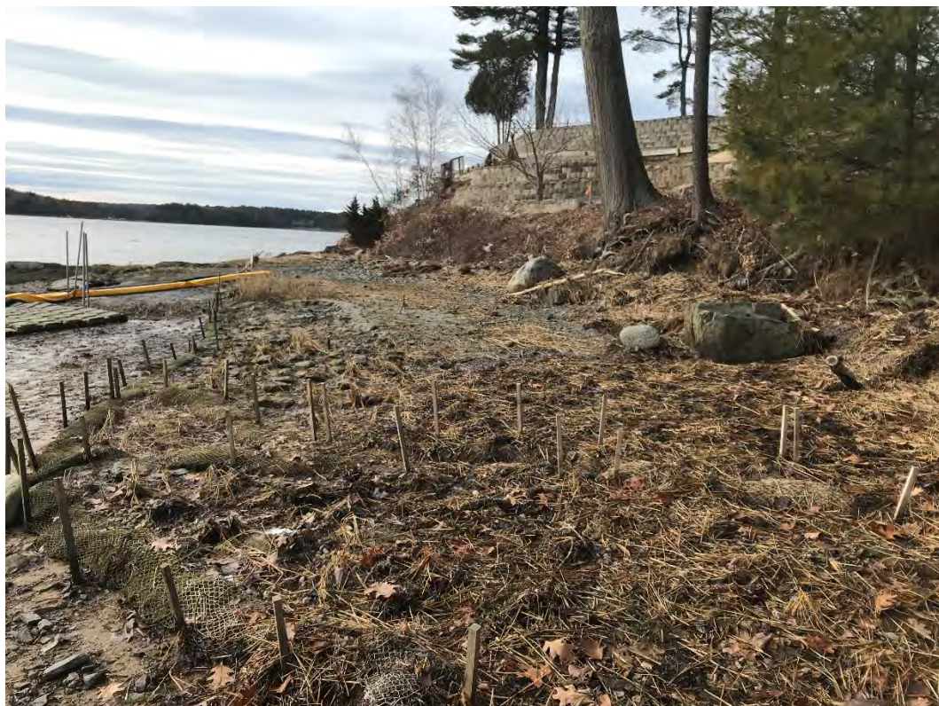
Fig 11: Salt marsh restoration at Gundalow Landing/east side of the bay. Viewing northwest. (01-19-21)
